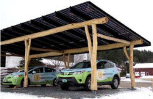
Round, unmilled timber might seem obsolete, but by using high-tech scanning and modeling, one company is bringing this form back into designers' repertoires at a cost that can compete with steel. And we're not just talking for a rustic log cabin aesthetic either: the company's fast-growing portfolio of projects includes contemporary designs at a high-end bakery, an industrial commercial building, and an outdoor pavilion.
